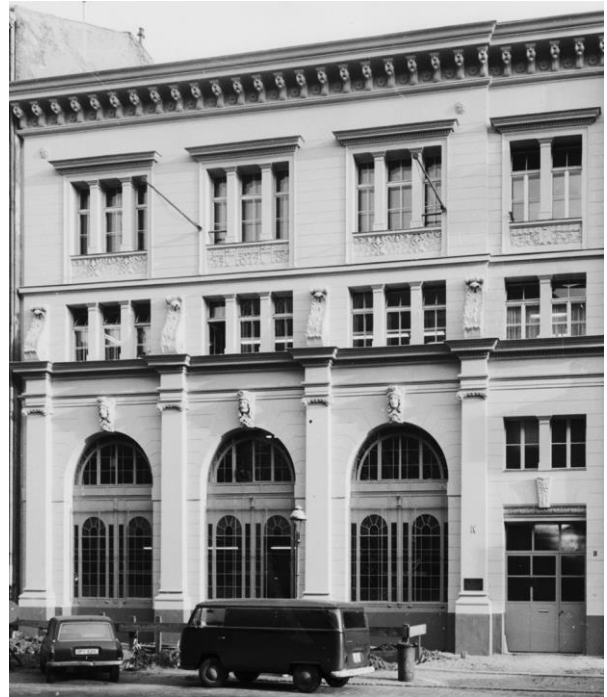
Fig. 5: The transformer station in Wilhelmshavener Strasse, built in 1900/01, was one of the first of its type in Berlin. The technical purpose of the building is difficult to recognise for the layman. (Source: Vattenfall Europe, Historical Archives, Berlin)
